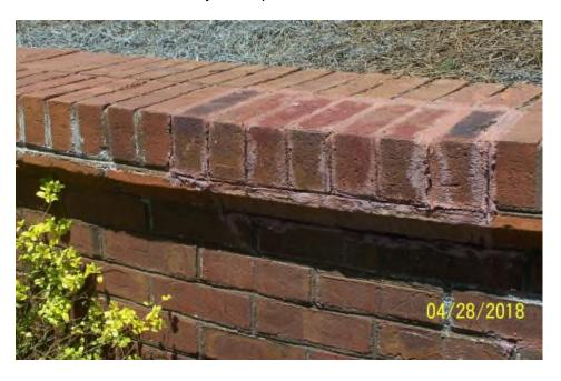
The repairs to the wall in the previous photo are not comparable to the original construction. A qualified mason is desirable because inexperienced workers will often perform work that is aesthetically undesirable.
