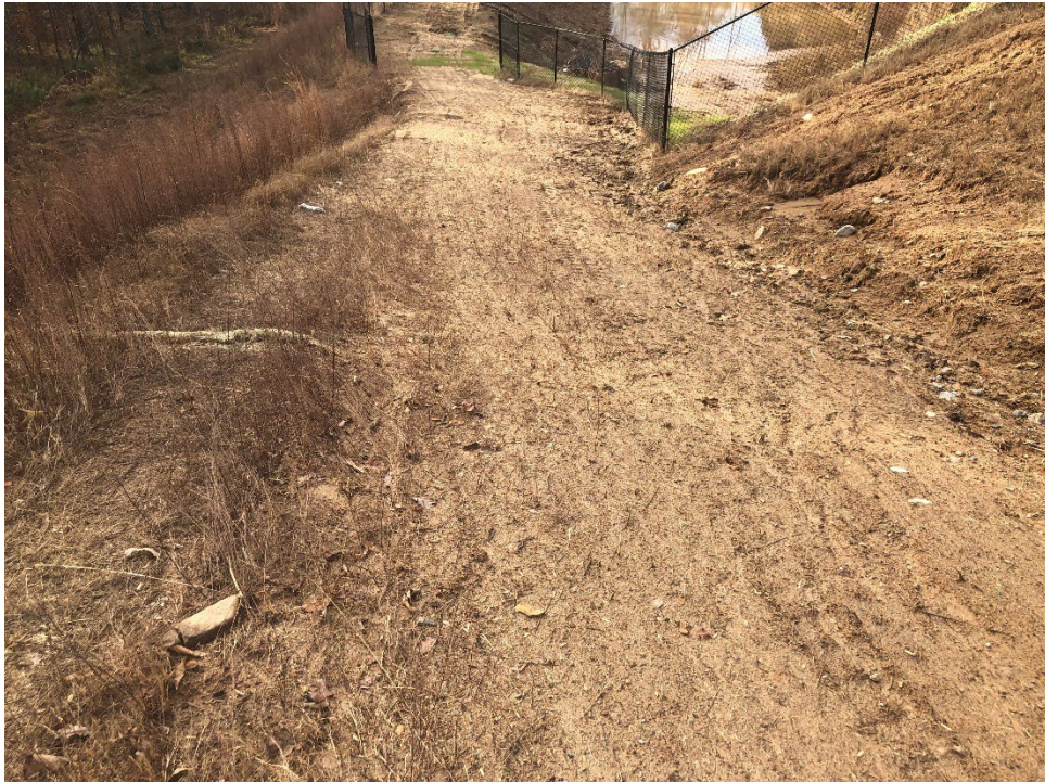
18. View of exposed soil at the maintenance road and slopes of the detention pond.
