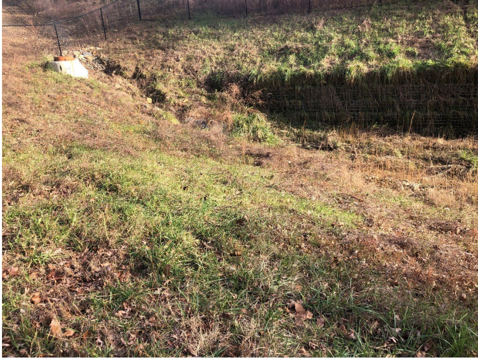
19. View of rill erosion from the maintenance road at the detention pond.
